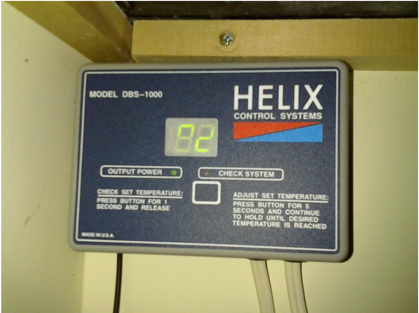
Figure 7. Helix ® DBS 1000 temperature control unit used to control Flexwatt Heat Tape ® .
